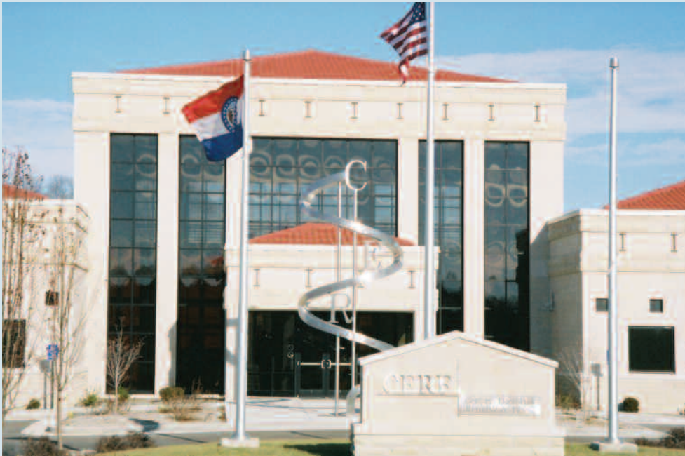
C&R fabricated the CERF sculpture for the County Employees Retirement Fund building in Jefferson City, MO
