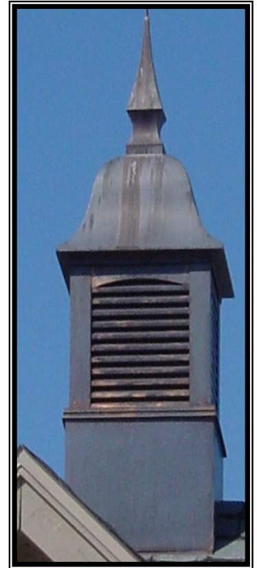
CR430-10-350 Petite Cupola with Square Base, Single Louvers & Bell Top w/ Finial Style CR350
